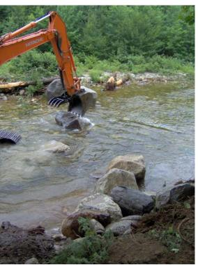
An excavator moves boulders into place July 22 to build a rock vane at the *Sunday River Outward Bound* Project in Newry. Rock vanes point upstream and deflect flows away from the eroding riverbank. Erosion at this location was so severe it threatened to undermine the nearby Sunday River Road.
